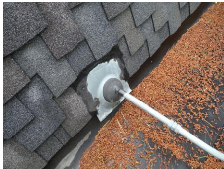
Improper flashing
